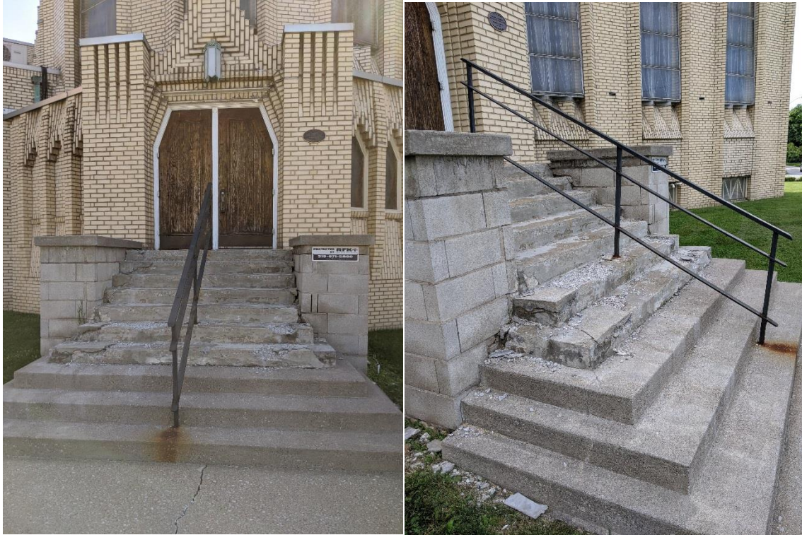
Previous appearance of deteriorated concrete condition at the Victoria Avenue Entrance
