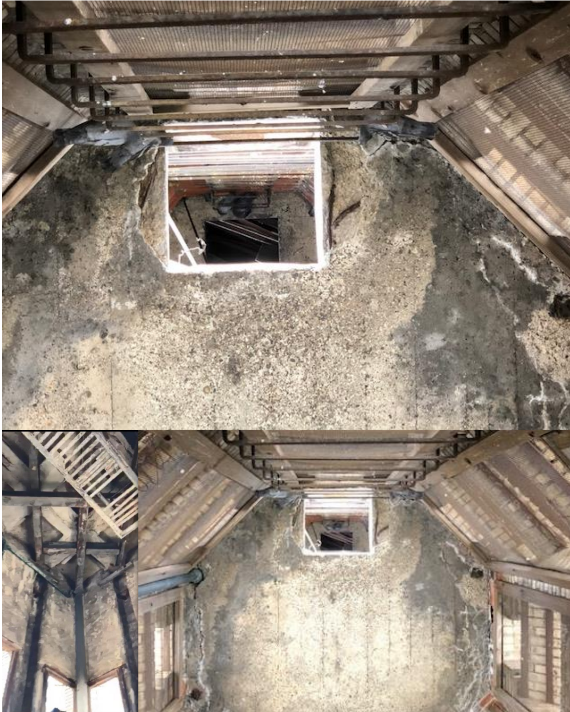
Condition and deterioration of Tower which shows visible cracking around the perimeter (not yet assessed by a structural engineer).
