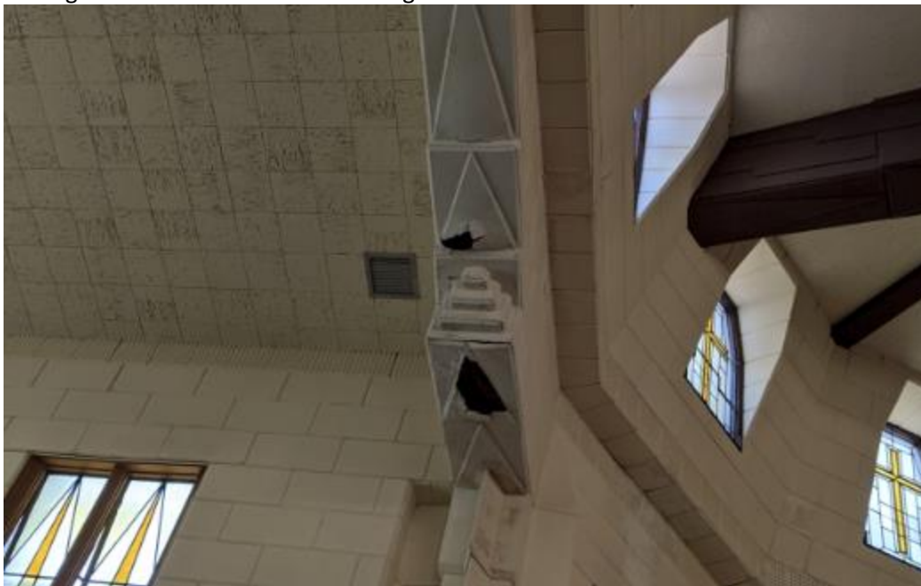
Damage to interior acoustical panels
