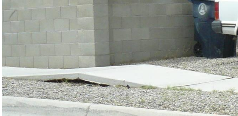
Fig. 4.2: Sidewalk Heaving/Buckling ( www.seeclickfix.com )
