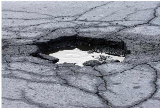
Fig. 4.3 Pothole in Asphalt Pavement ( pavenow.net )
