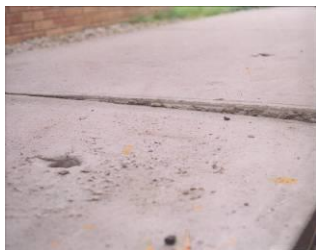
Fig. 8.1a: Sidewalk Uplift Repaired by Mudjacking ( www.mudjacking.com )
