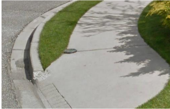
Fig. 6.2a: Water Valve in Sidewalk (WUC) ( Google Maps - ©2013 Google)
