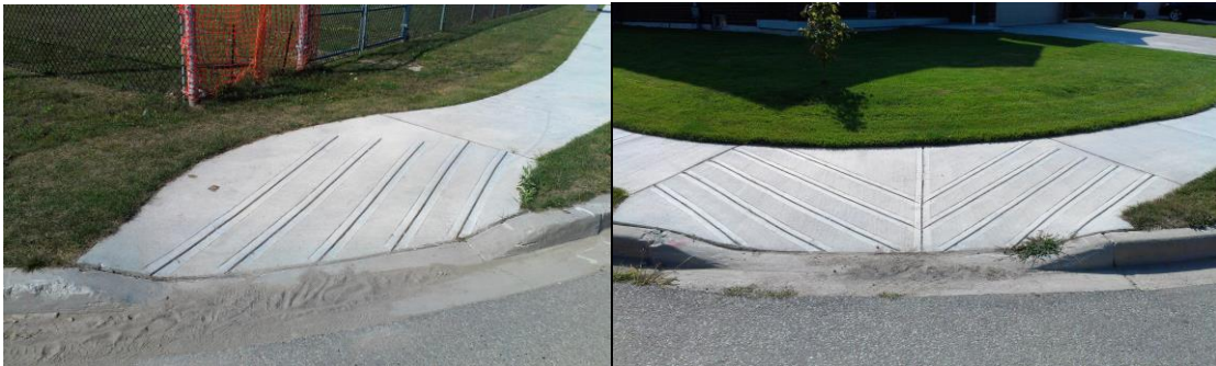
Fig. 3.6c: Wheel Chair Ramp with control joints as stamping (City of Windsor - IMS Photo)
