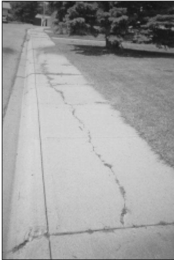
Fig. 4.1.2: Longitudinal Cracking of Concrete ( http://irc.nrc-cnrc.gc.ca )
