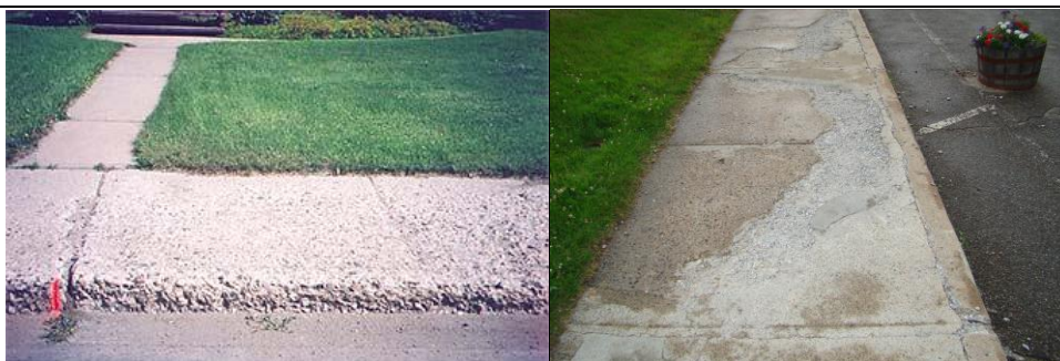
Fig. 5.3: Spalling of a Concrete Sidewalk ( www.rss.ca , www.concretesealerandblanket.org )
