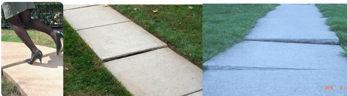
Fig. 4.5.1: Uplifting of Concrete ( http://vtconcretecutting.com , www.pccconcrete.com )
