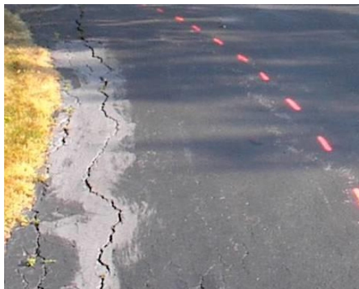
Fig. 4.1.5: Edge Cracking of Asphalt ( www.asphaltrestore.com )
