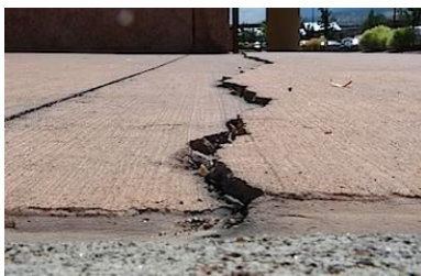
Fig. 4.6: Displaced Panels at a Crack ( www.nachi.org )
