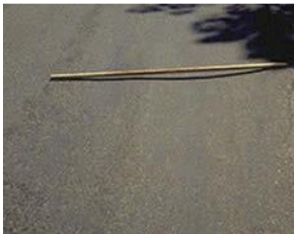
Fig. 4.4 Rutting in Asphalt ( halifax.ca )
