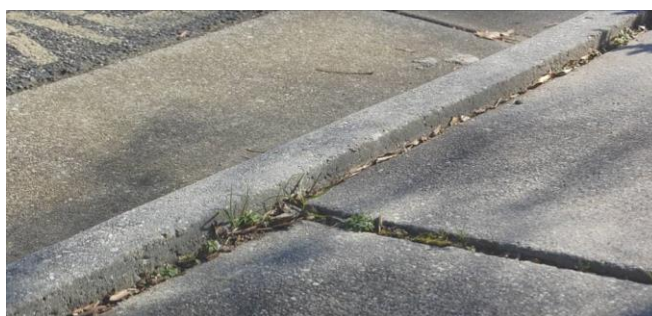
Fig. 4.8 Settled Sidewalk Panels Along Back of Curb ( concretejack.com )
