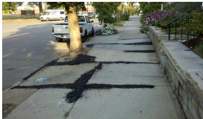
Fig. 8.3: Asphalt Patches on Sidewalk ( www.chpn.net )
