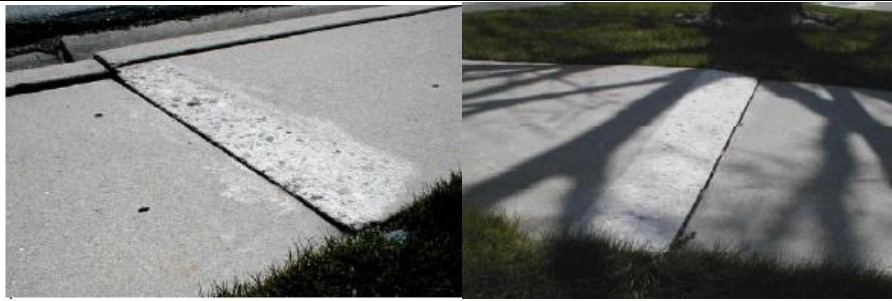
Fig. 8.2: Examples of Uplifts Repaired by Grinding (left) and Saw Cutting (right) ( http://service.govdelivery.com )
