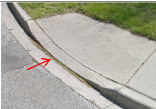
Fig. 3.6e: Wheel Chair Ramp with Lip at Curb in Gutter Pan and no stamp ( Google Maps - ©2013 Google)
