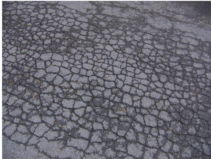
Fig. 4.1.4: Alligator Cracking of Asphalt ( http://toheroa-jim.blogspot.ca )
