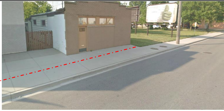
Fig. 3.2g: Shows Area to be Inspected Between Control Joint (Red Line) and Curb ( Google Maps - ©2013 Google)
