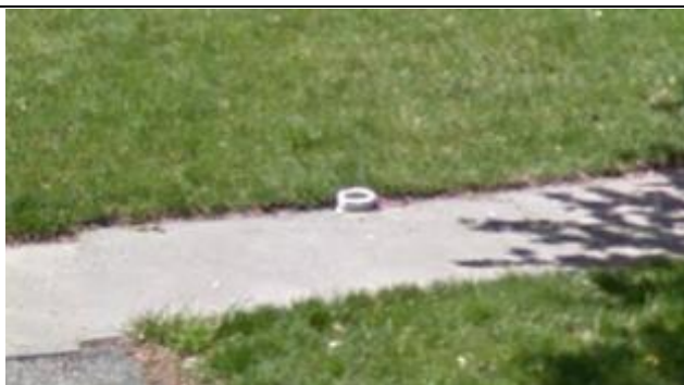
Fig. 6.3: Sewer Cleanout in Sidewalk ( Google Maps - ©2013 Google)
