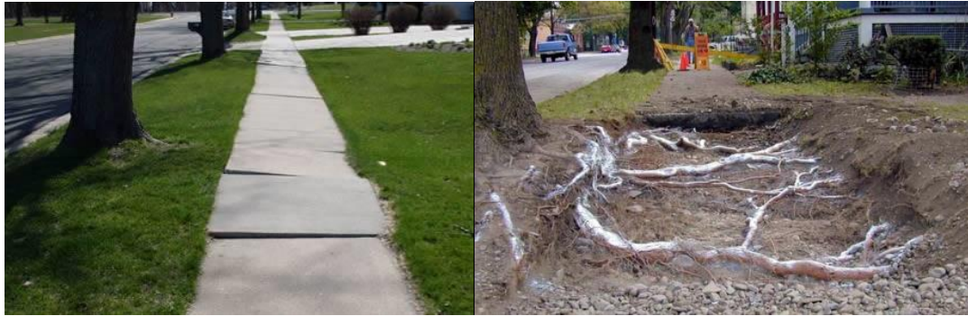
Fig. 5.1: Uplifting Caused by Tree Roots ( www.ci.middleton.wi.us , www.oneilstreeservice.com )
