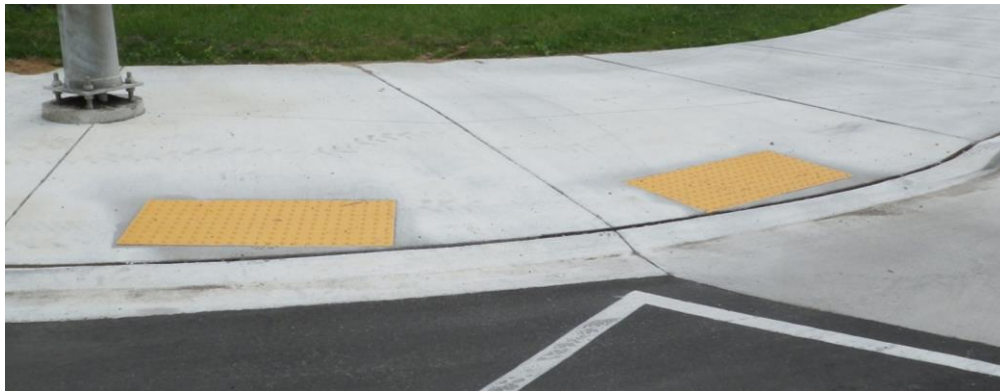
Fig. 3.6d: Wheel Chair Ramp with Pedestrian Warning Plates (Tactile Dome) (City of Windsor - IMS Photo)
