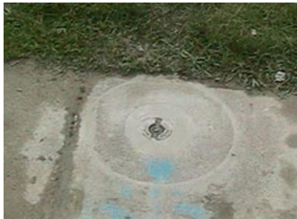
Fig. 6.2c: Curb Stop (WUC) Present in Sidewalk ( www.utilitor.ca )
