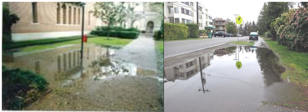
Fig. 4.7: Drainage Problems on Sidewalks ( www.owl.net.rice.edu , www.daily.sightline.org )
