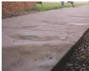
Fig. 8.1a: Sidewalk Uplift Repaired by Mudjacking ( www.mudjacking.com )
