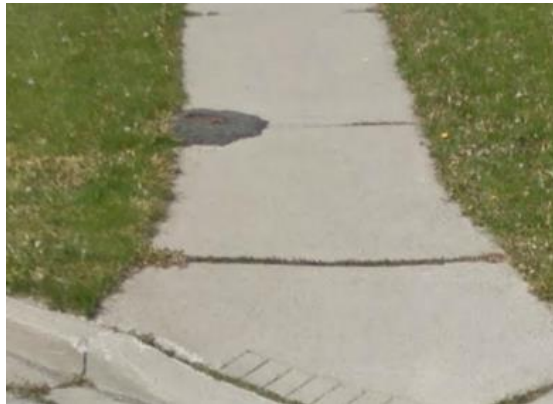
Fig. 6.2b: Water Valve (WUC) in Sidewalk with Asphalt Patch ( Google Maps - ©2013 Google)
