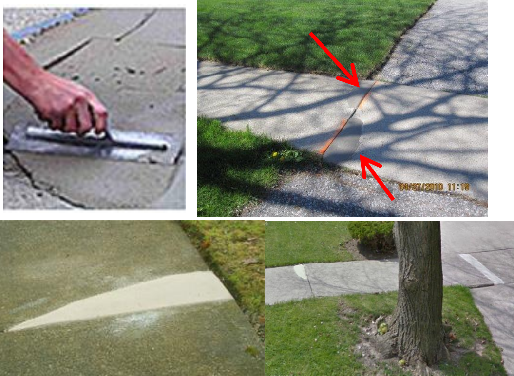
Fig. 8.4 MG-Krete Ramping/Patching ( vancouver.ca ), ( northlandconstruction.com ), ( vancouver.ca ), ( Google Maps - ©2013 Google)
